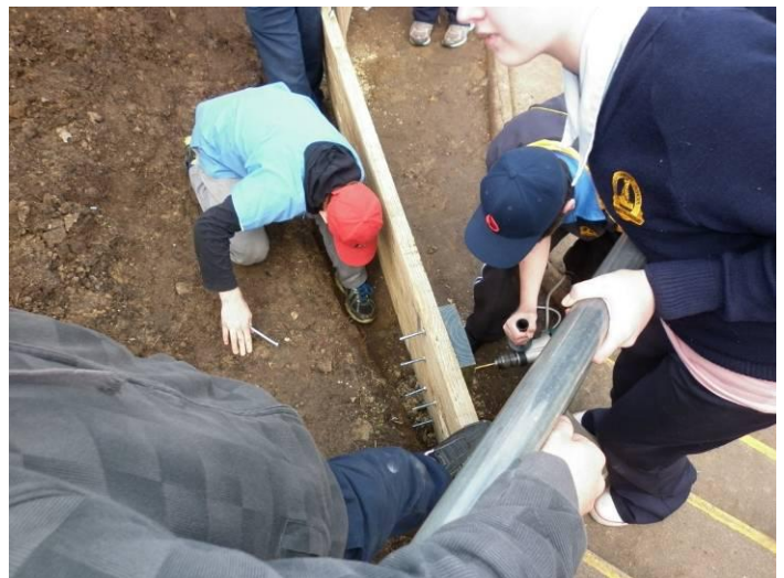
Students building the retaining wall.
